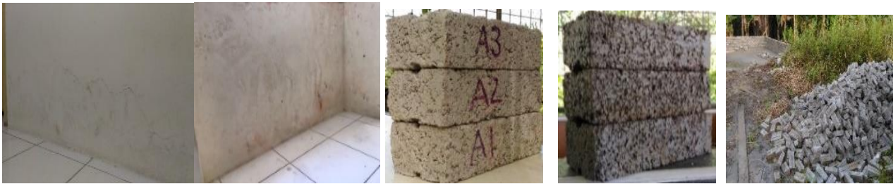
Figure 1(a). Condition of Wall Surfaces
