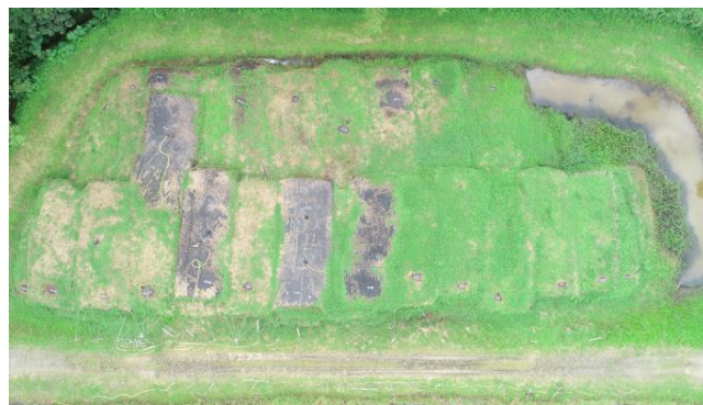
(b) Backlog of sludge nearby the pond
