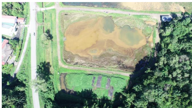
(a) Accumulated sludge in the treatment pond
